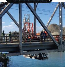
This is a 13m Moog platform mounted on tracks. It's incredibly light and narrow making it perfect for narrow bridges requiring a light load. This unit has the option to come with or without an operator and we can deliver it to anywhere in Australia.
